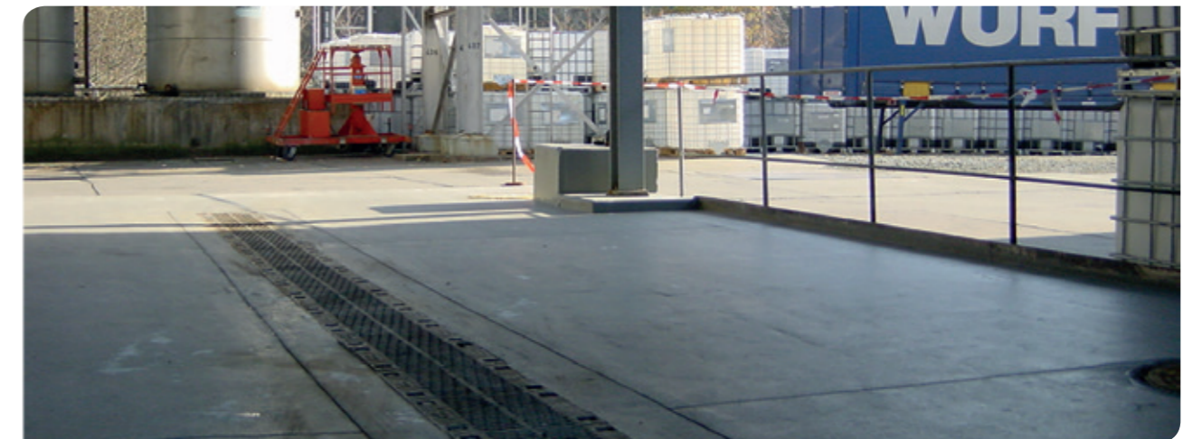
Picture 4: Floor coating of a truck-wash station in a chemical plant
